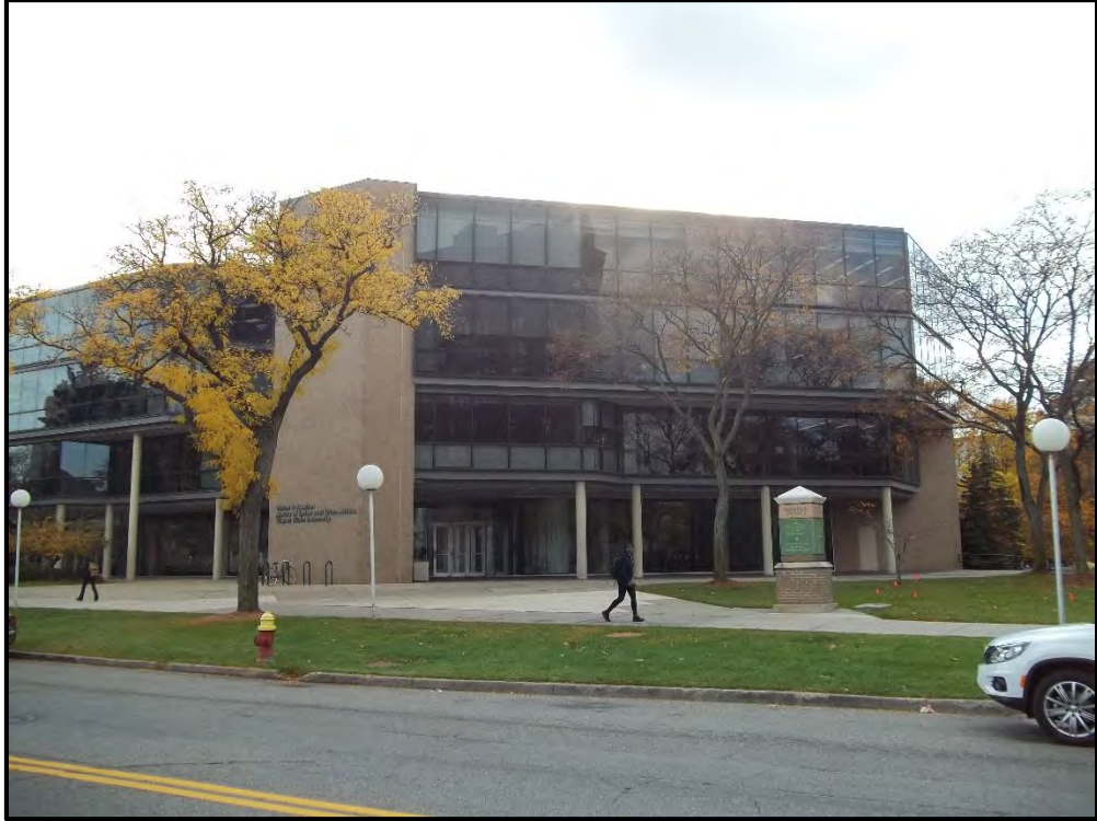
East and North Facades
